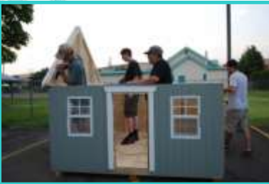
EPIC employees and friends building the Gingerbread Cottage.
